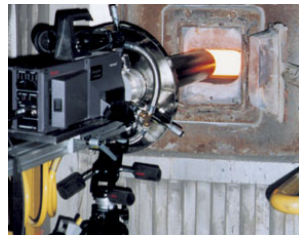
Special high temperature vortex tubes keep a boroscope lens cool while inserted into a 1200°F (650°C) boiler porthole.
